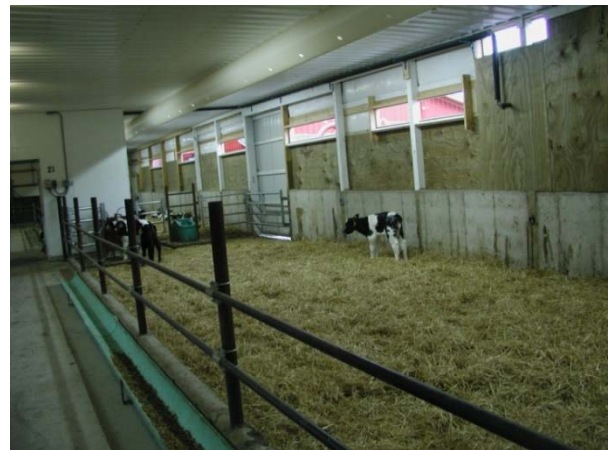
Calf barn with computerized calf feeder and tube ventilation
