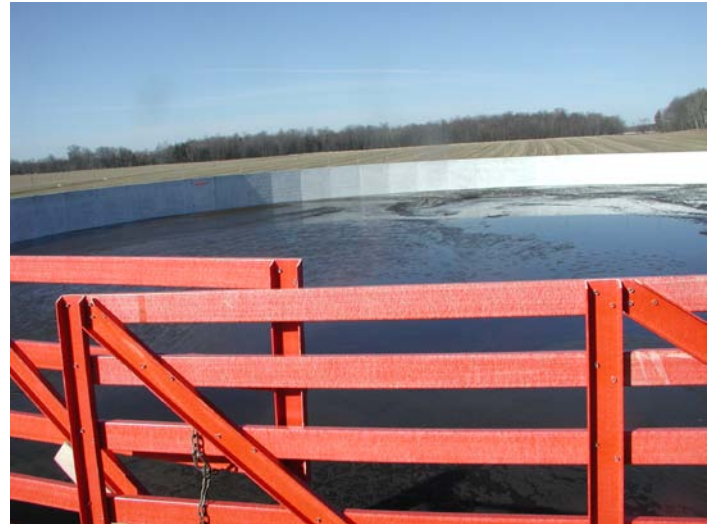
Concrete lined manure storage.
